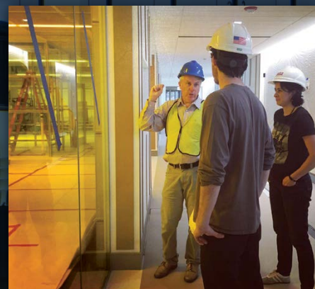
Peter Duda, Technical Manager of the Pritzker Nanofabrication Facility, explains the cleanroom capabilities to IME researchers during the final stages of construction in the summer of 2015.
